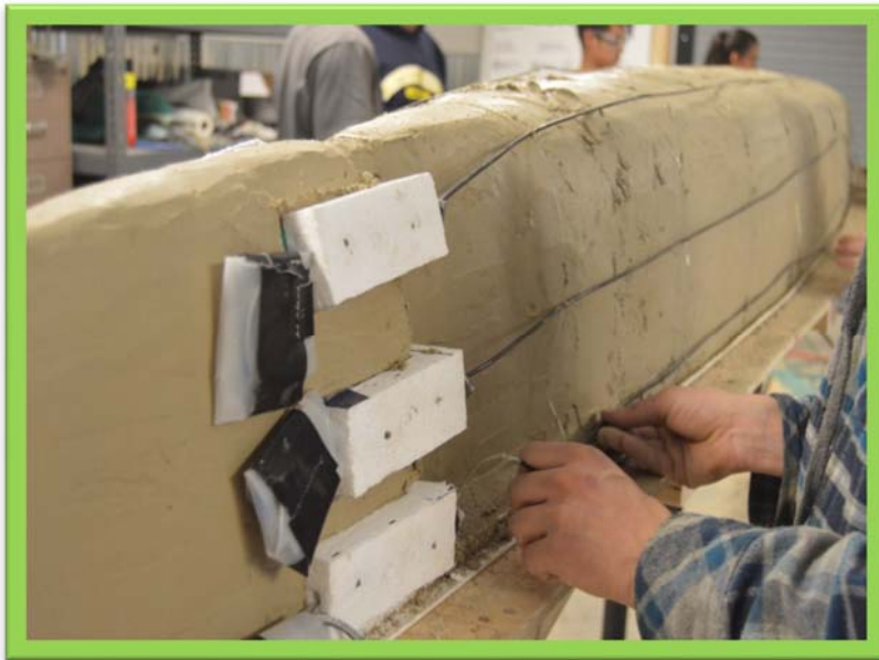
Figure 14: Post Tensioning System During Casting
