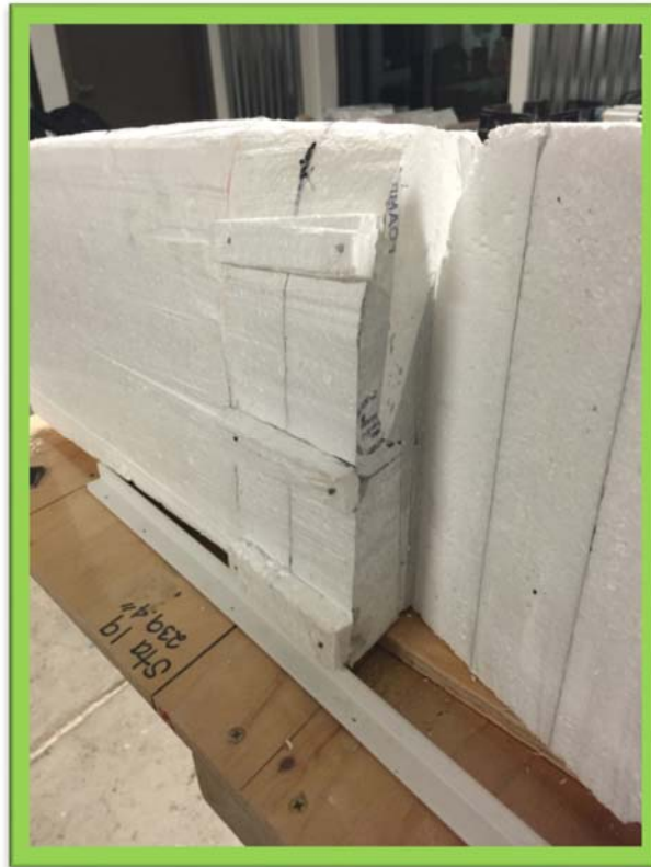
Figure 7: Cut Out of Bulkhead for Post Tensioning Anchorage
