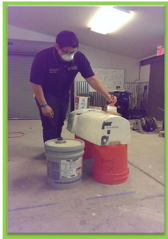
Figure 8: Application of Form Release Oil
