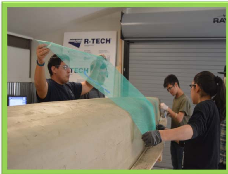
Figure 12: Placing of Reinforcement
