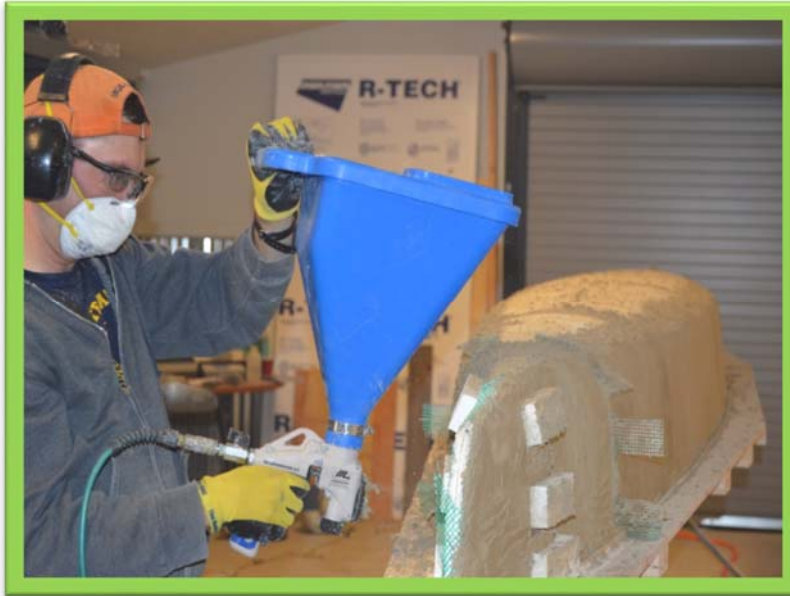
Figure 11: Placing Concrete Using Spray Method
