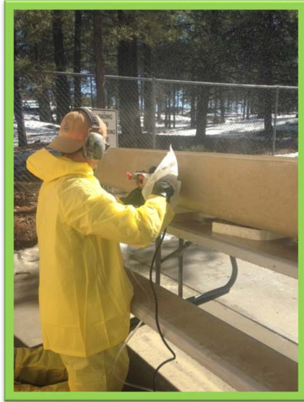
Figure 17: Finishing - Sanding
