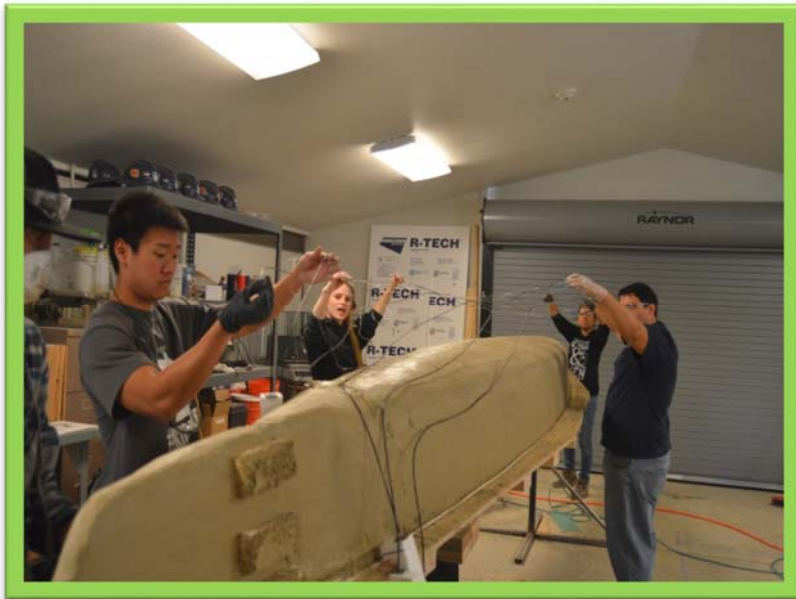
Figure 13: Placing the Post Tensioning Cables Net
